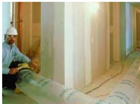
Drywall installation went quickly as joint compound dried in hours.
