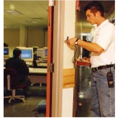
Computer centers were kept in use upstairs as drying continued downstairs.
