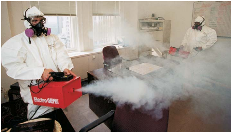
Chemical agents were used to "fog" interior space, neutralizing the smell of smoke.
