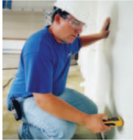
Munters measures moisture content of structural materials to determine if drying is thorough.
