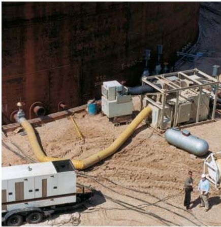
Set up outside the tank, Munters gas reactivated dehumidifiers reduced fuel costs, while providing dry air that sped the process by allowing continuous work and faster curing of the coating.
