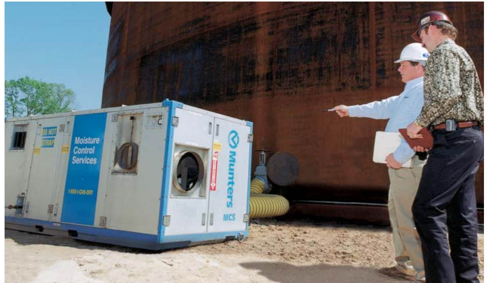
Set up outside the tank, Munters gas reactivated dehumidifiers reduced fuel costs, while providing dry air that sped the process by allowing continuous work and faster curing of the coating.
