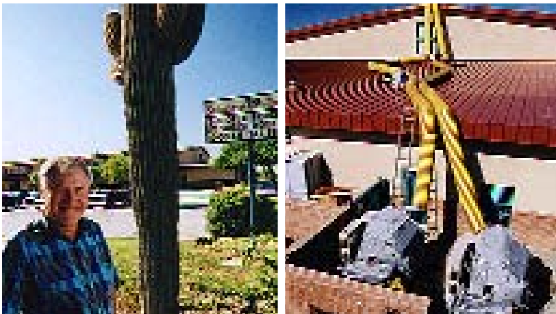
Above left: Jim Sherman, safety and loss coordinator for the Peoria School District, said the entire roof was in jeopardy. "If drying didn't work out, reconstruction would have cost the school $750,000. To leave it wet would have subjected the school to serious mold and mildew problems." Above right: Two HC-4500 dehumidifiers were used to generate the dry air needed to complete the project.
